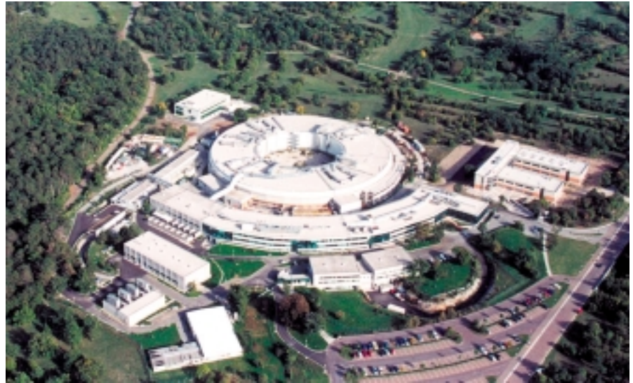
Figure 1. The ELETTRA facility in Trieste, Italy (Courtesy of ELETTRA).
